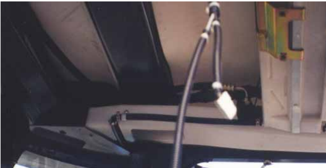
Evaporator hoses running back around back of cab headliner area.
