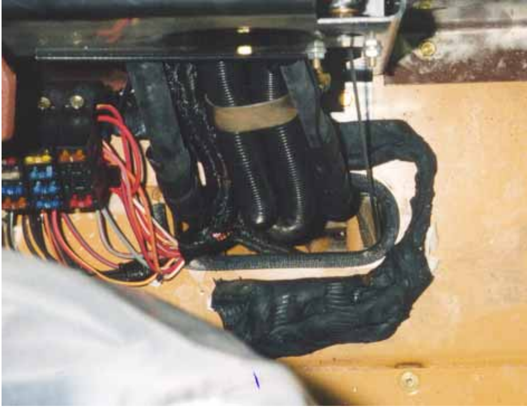
Hoses routed through floor of cab.
